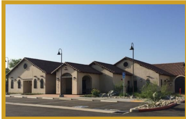
Merrill Center Crisis Stabilization Unit (CSU) 14677 Merrill Avenue, Fontana (951) 643-2340
