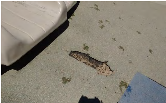
Torn Mat at Bottom of Slide
