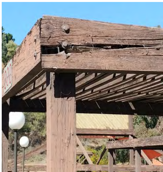
Pool Area Shade Cover with Split Support Beam
