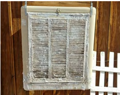
Minerals on Evaporative cooler
