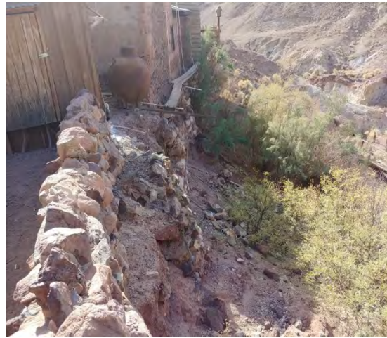
Eroded Building Foundation
