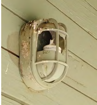
Broken Light Fixture
