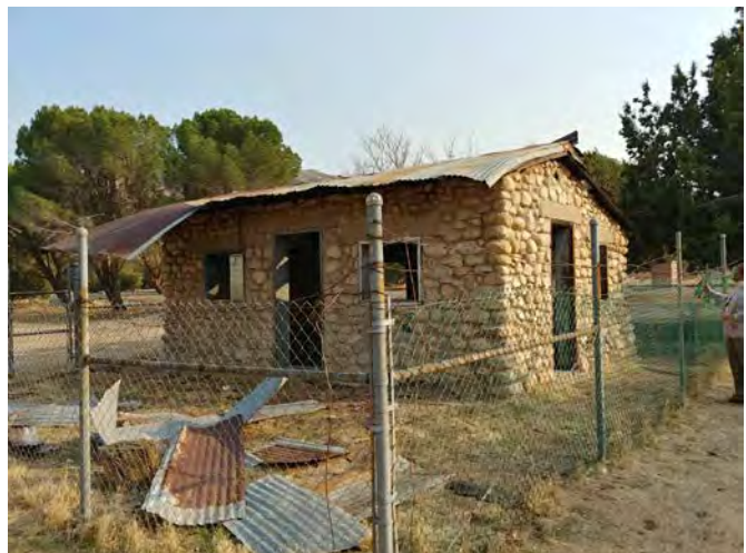
Rock Building with Roof Damage
