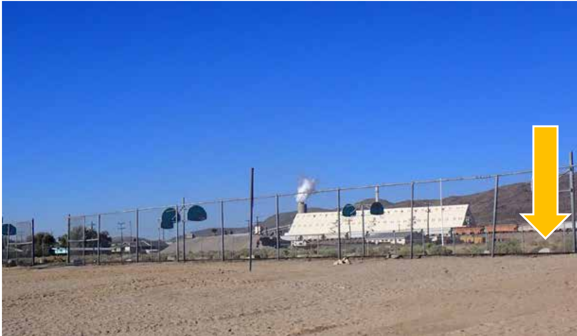
New Highschool Site (Photo Taken 09/05/2023)
